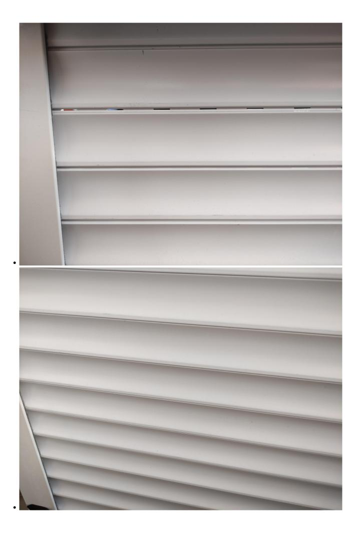
Figure 4. Example of roller shutter setup: left - with "clearance", right - fully closed.
